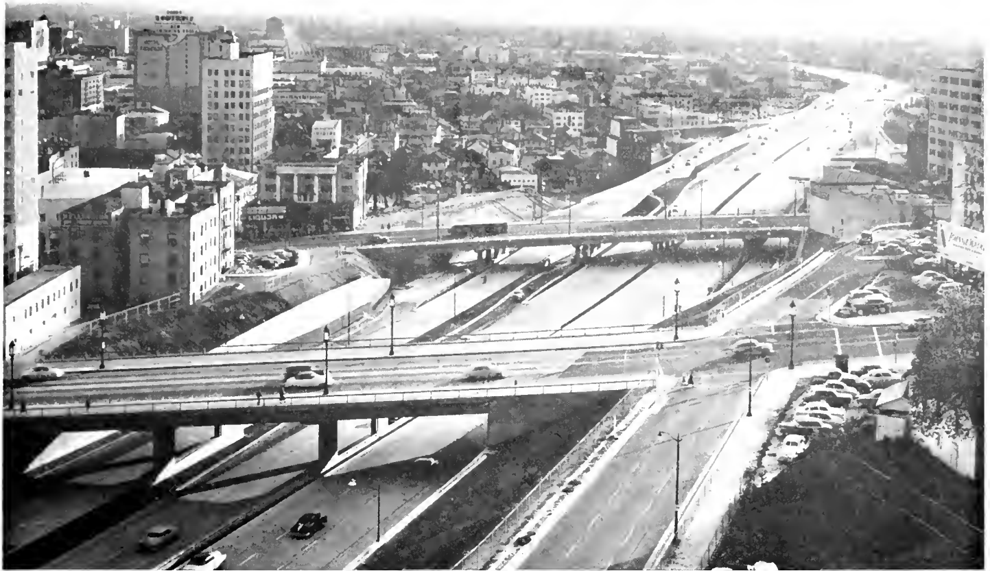
Looking south along Harbor Freeway. Wilshire Boulevard Overcrossing in foreground; Seventh Street Overcrossing in center.
